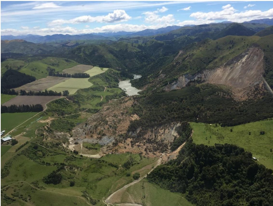
Figure 6: Landslide dam on the Leader River shortly after the earthquake. The landslide is a slump/block slide in a siltstone unit and is characteristic of the large landslides in weak Neogene rocks. The landslide dam overtopped and partially breached on the 13-14 February 2017 (Environment Canterbury).
