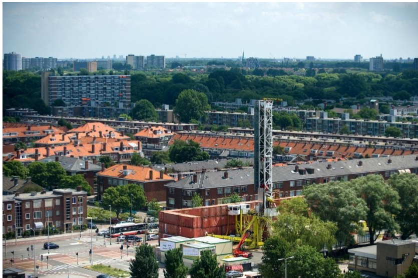
Drilling in Central The Hague
