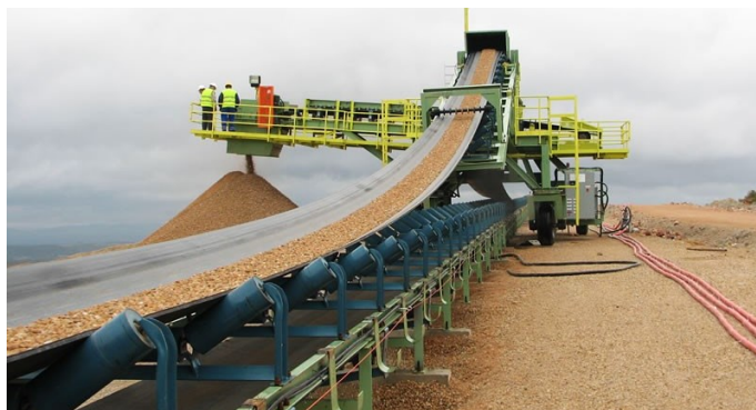
Figure 2-26: Lifting and unloading a conveyor belt with a belt tripper [236]
