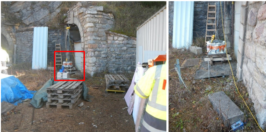
Figure 230: Blast set-up used in blast test 1.
