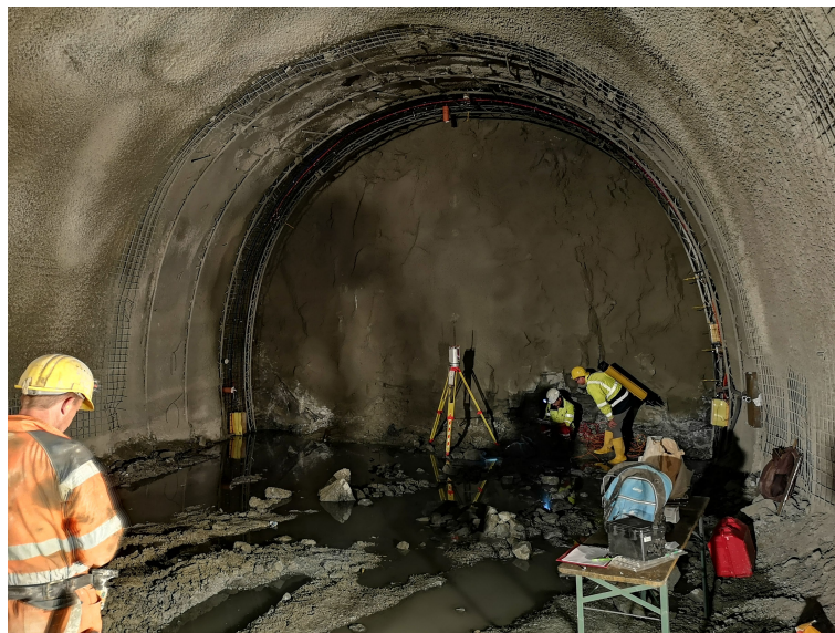
Fig. 4.1 Conditions at a tunnelling construction site at the working face.
