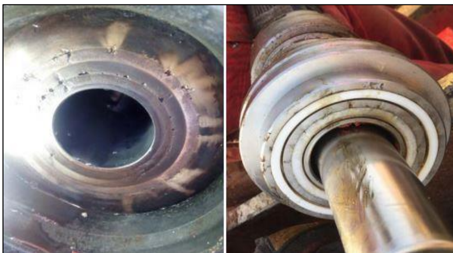
Figure 22: Washed out stuffing box.
