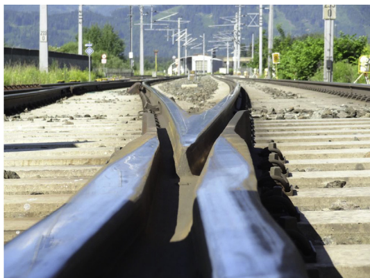
Fig. 1. A deformed manganese crossing in track.
