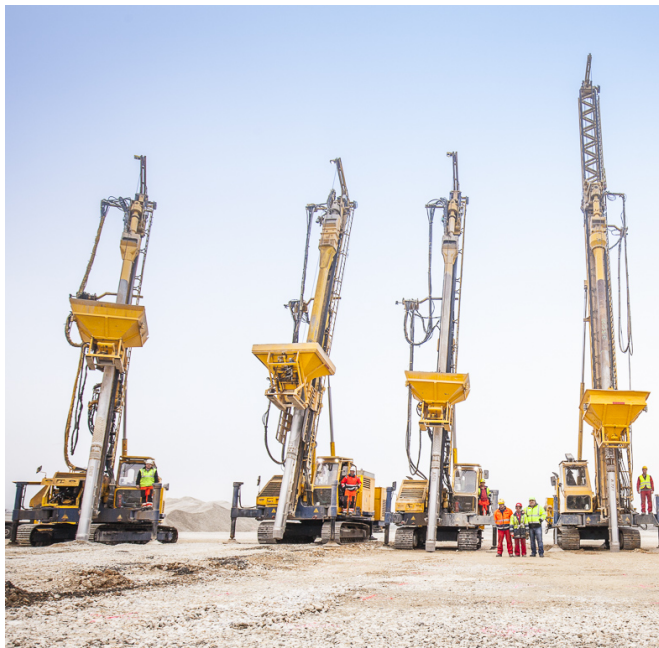
(a) Vibrocats (Courtesy of Keller)
