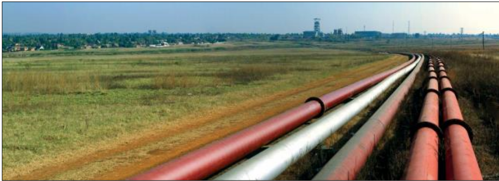
Figure 48. DRDGOLD transportation of tailings by pipeline system (DRDGOLD, 2018).
