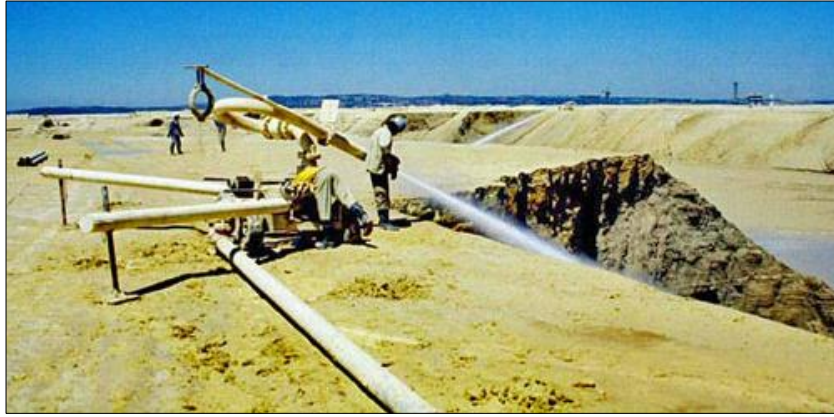
Figure 55. Hydraulic exploitation of tailings from the top (Engels, 2017).
