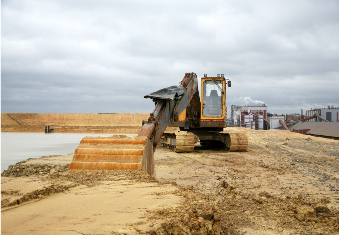
Figure 14: Building a containment dam from jarosite (Sensitive source)
