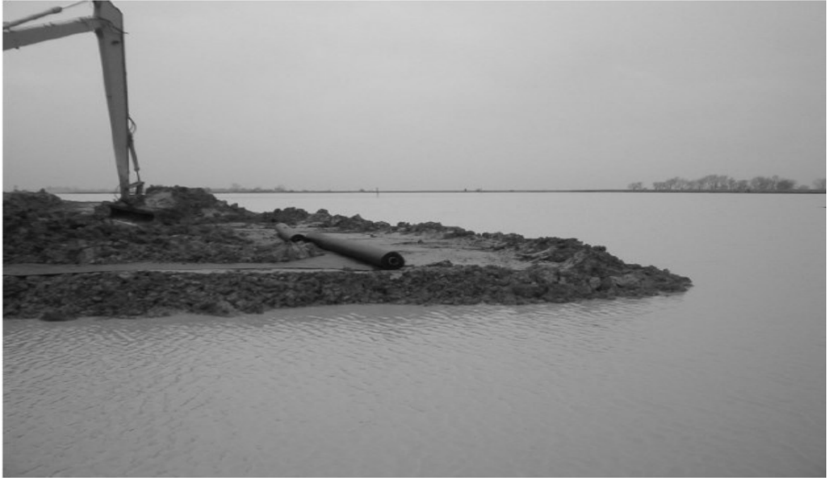
Figure 12: Transition from jarosite to jarofix disposal; Appliance of geo-textile (Zöller, 2012)
