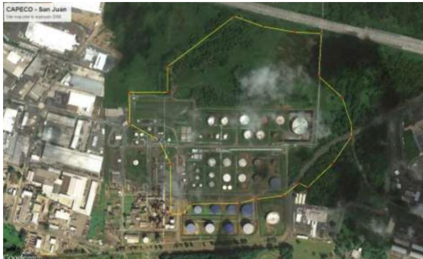
Figure 32: CAPECO site with marked area of the vapour cloud [18] p. 123
