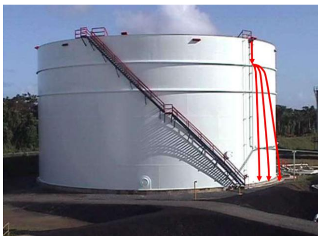
Figure 31: Tank geometry and suggested trajectories of over spilled gasoline [18] p. 126
