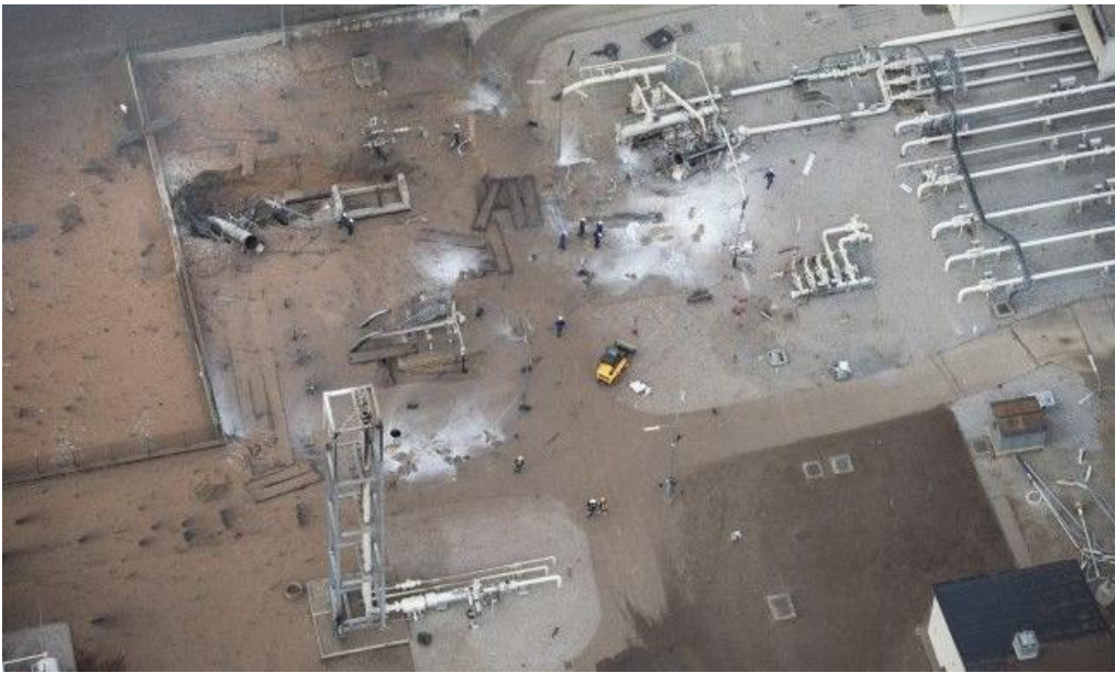
Figure 16: Aerial view of the area of the accident after the fires were extinguished [31]
