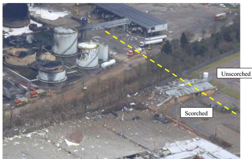
Figure 29: The edge of the vapour cloud marked by scorching and blast damage [18] p. 53
