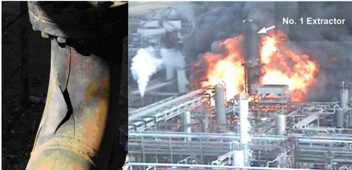
Figure 19: Crack in the 10" propane pipe and the site 90 seconds after ignition (CCTV) [11] p. 23+16
