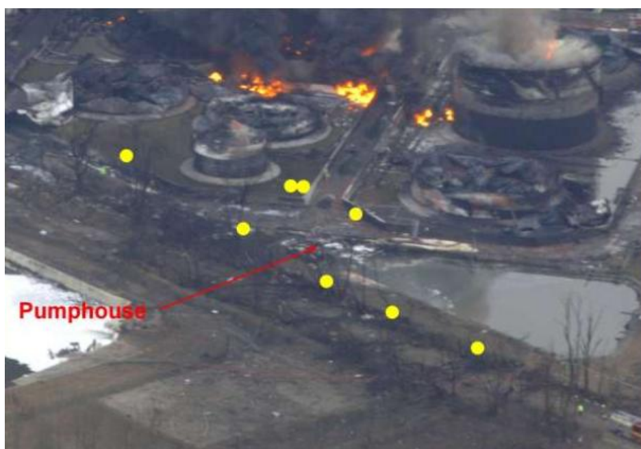
Figure 26: Burning tanks and pump-house marked [18] p. 60
