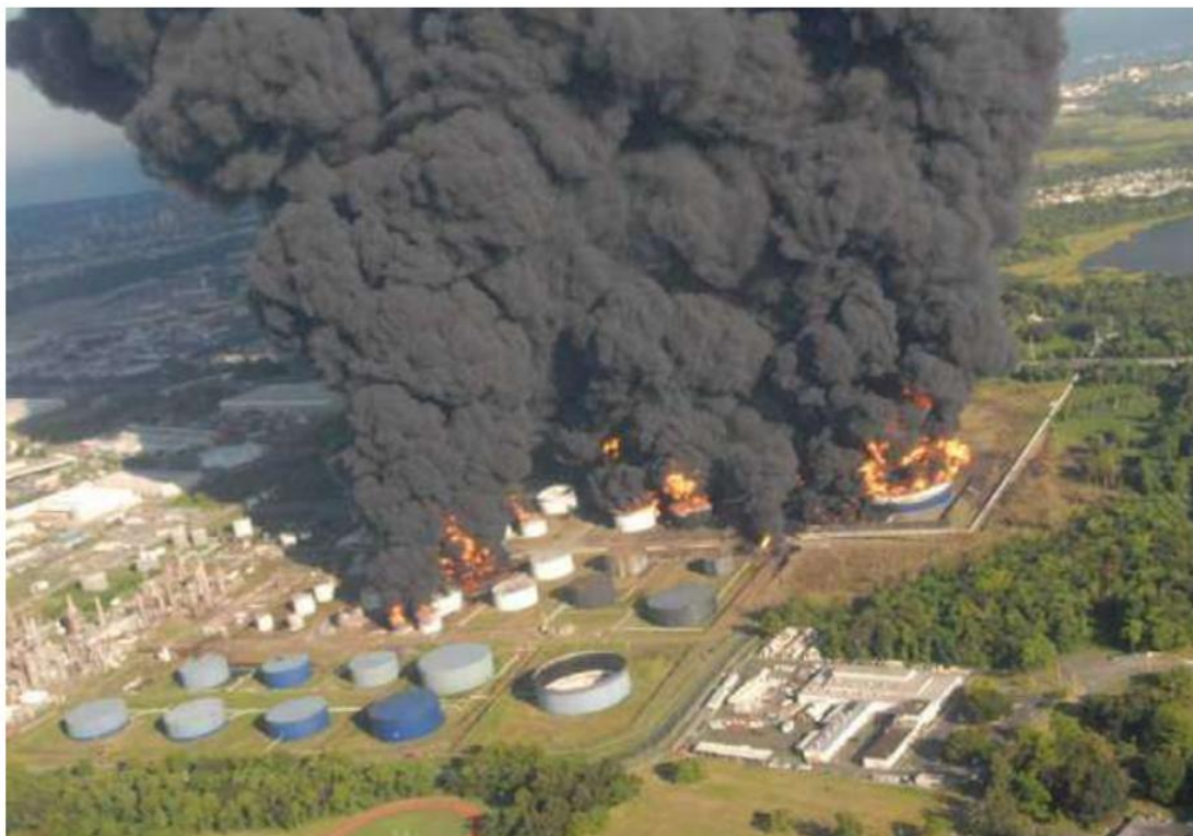
Figure 30: Multiple tank fires at the CAPECO gasoline terminal in San Juan [4] p. 24
