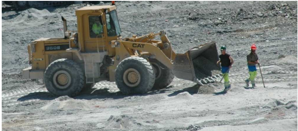
Figure 6.5: Stemming of boreholes after charging via wheel loader's assistance
