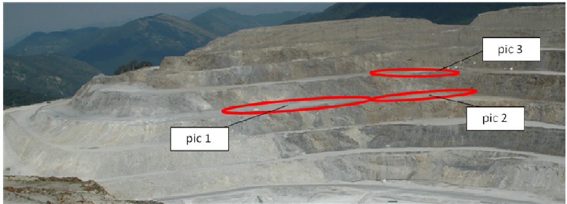
Figure 11.4: Overview back break on bloc 3 (pic 1 or Fig. 11.6 and pic 2 or Fig. 11.7) and bloc 4 (pic 3 or Fig. 11.8)
