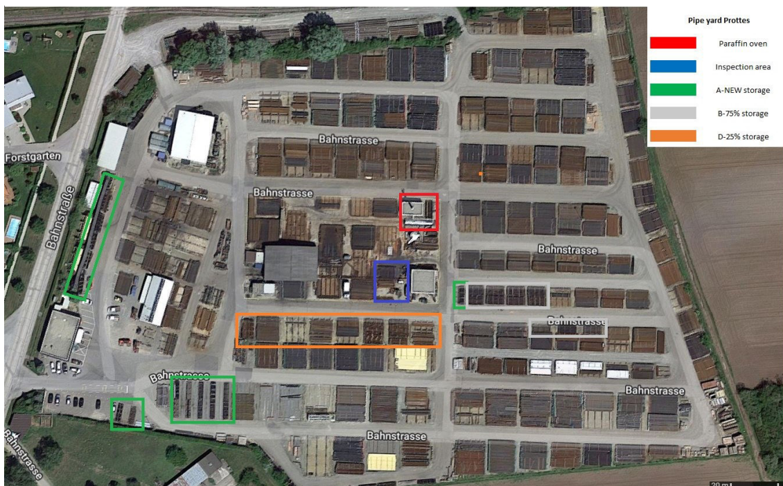
Figure 24: Pipe yard in Prottes
