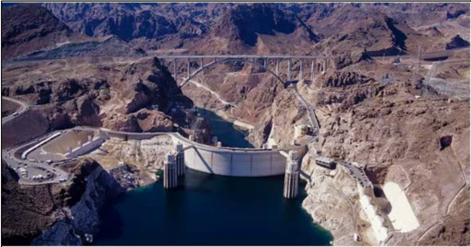
Figure 6. Hoover Dam on the Colorado River. Source: [National Park Service]( https://www.nps.gov/lake/learn/historyculture/hoover-and-davis-dams.htm )
