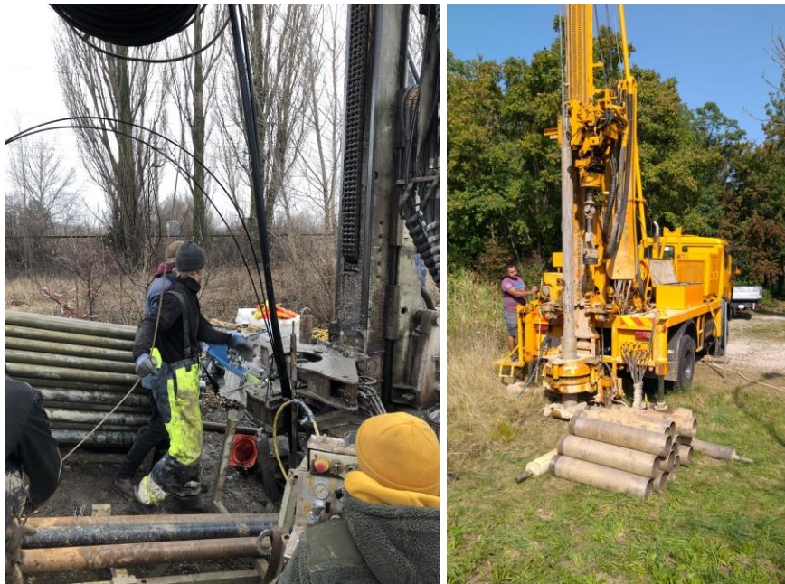
Figure 7: 150 m flush drilling (left) and 30 m core drilling (right) drilled at the site of the NÖM plant in spring and autumn 2020
