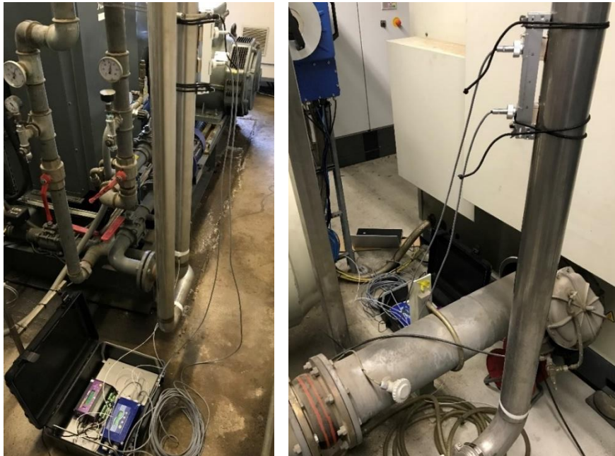
Figure 33: Measurements on the HDD systems: Atlas Copco (left) - LMF (right)
