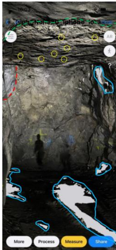
Figure 27: Highlighted details of the model generated with the iPhone 12 Pro, using the 3DScannerApp. The green dotted line represents the transition from shotcrete to exposed rock; the red dotted line highlights the transition from exposed massive sulphide to exposed shales; the yellow circles indicate the position of the detected expansive bolts and the areas highlighted in blue are the areas that the device was unable to capture and thus correctly generate a model.
