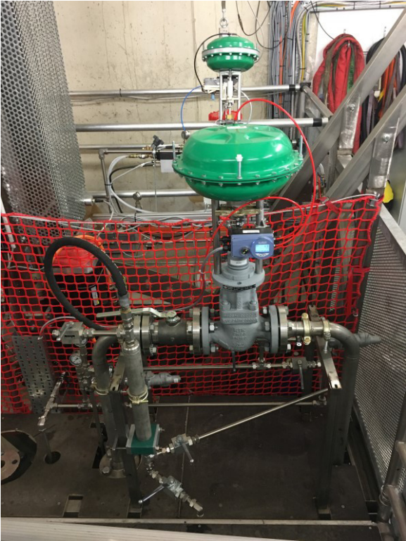
Figure 61: Pneumatic regulating valve and sampling device
