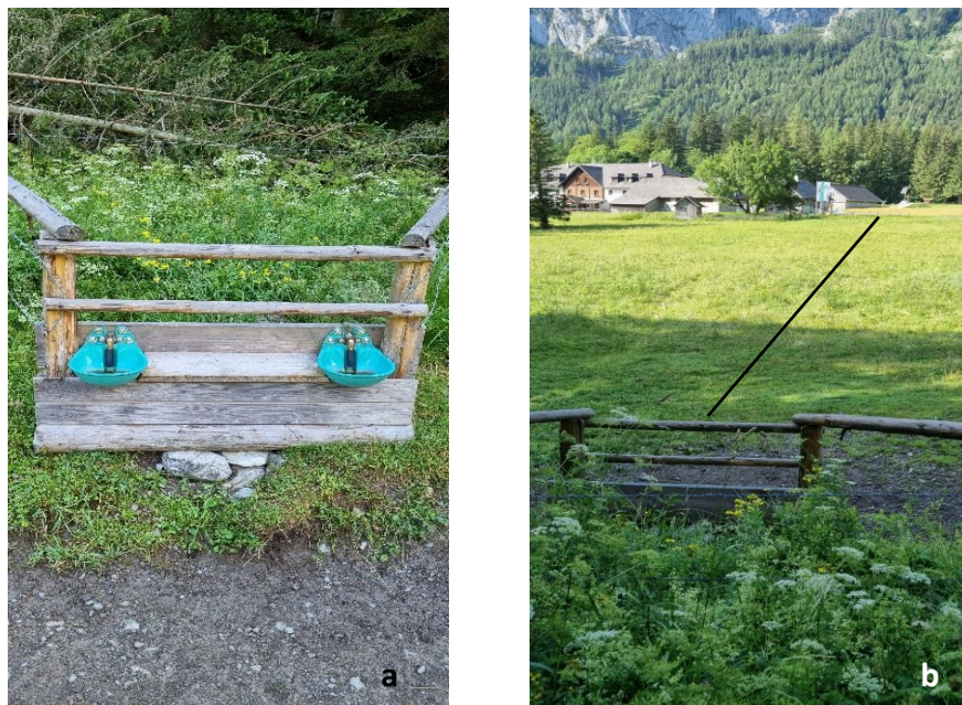
Figure 40: (a) Cattle trough whose underground pipe creates an anomaly - front view. (b) View from behind the cattle trough to visualize the course of the pipe (black line).
