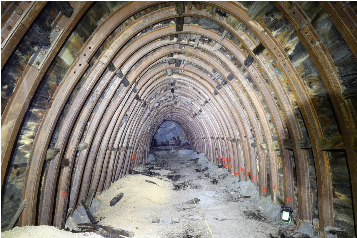
Figure 71: Detailed picture of the arches 60 to 70.
