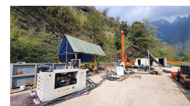
Figure 1: The drill site an early phase of the drilling operation.
