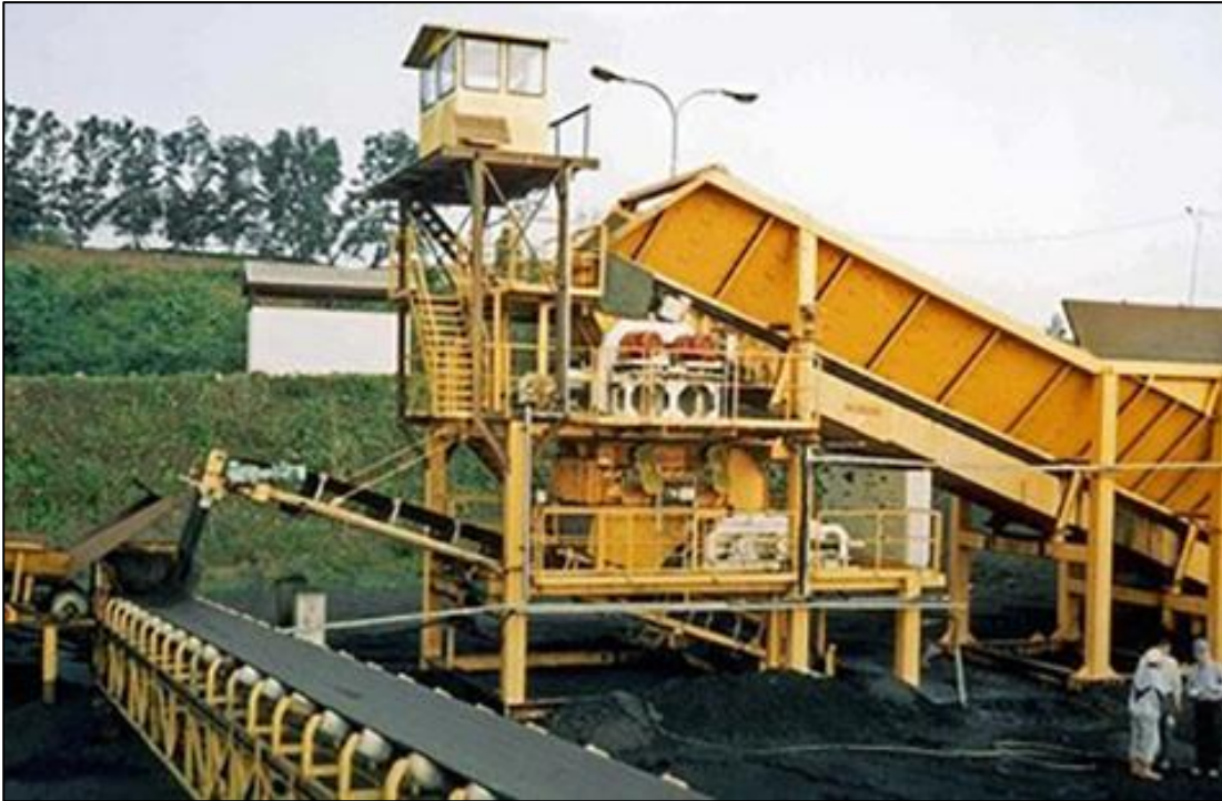
Figure 9: Fixed In-Pit Crusher Station of FLSmidth [5]
