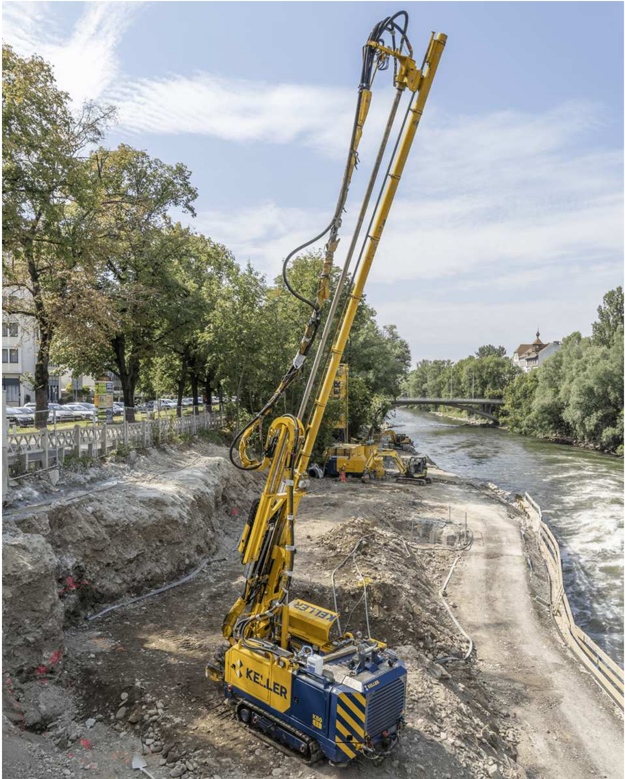
Figure 1: Rig in operation during the drilling of test holes for the acquisition of representative data. This should also verify the sensor's capability to survive the harsh environment during drilling.
