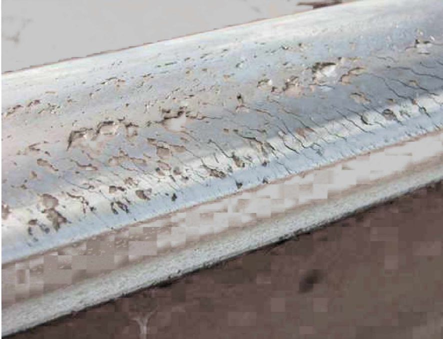
Figure 5.7.: Spalling and Head Checks on a badly worn rail head. Photo by voestalpine.
