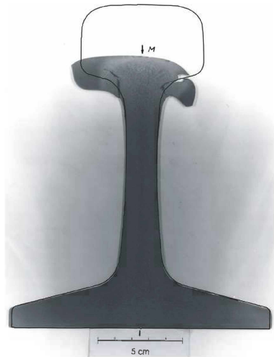
Figure 5.4.: Example of worn rail in heavy haul operations. Photo by voestalpine.
