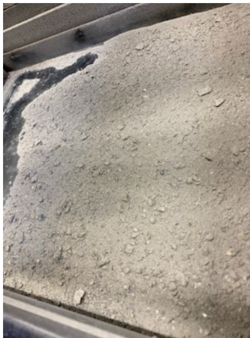
Figure 4.30: Debris of B20 concrete sample
