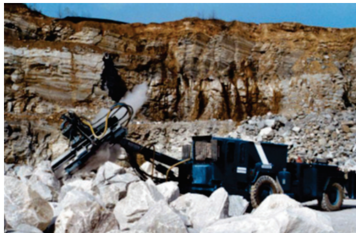
Figure A.40: Plasma blasting rock breaker unit [208]
