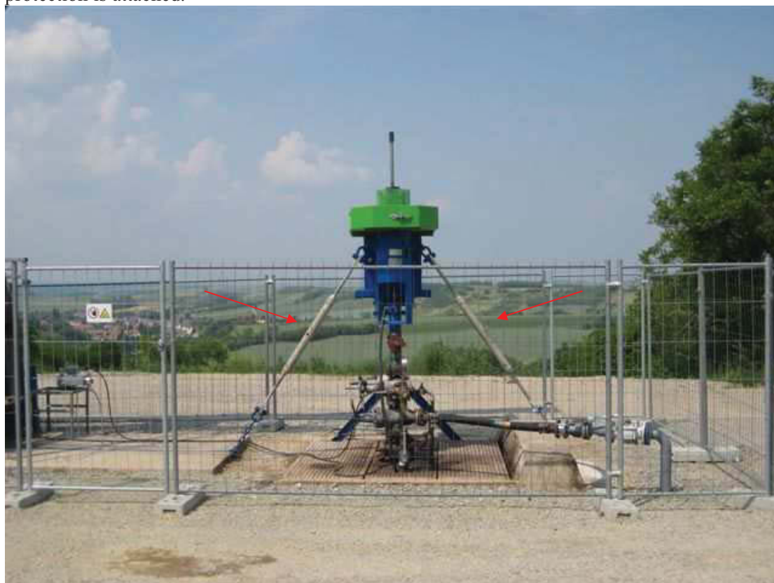
Figure 53 protection against vibrations of DH.
