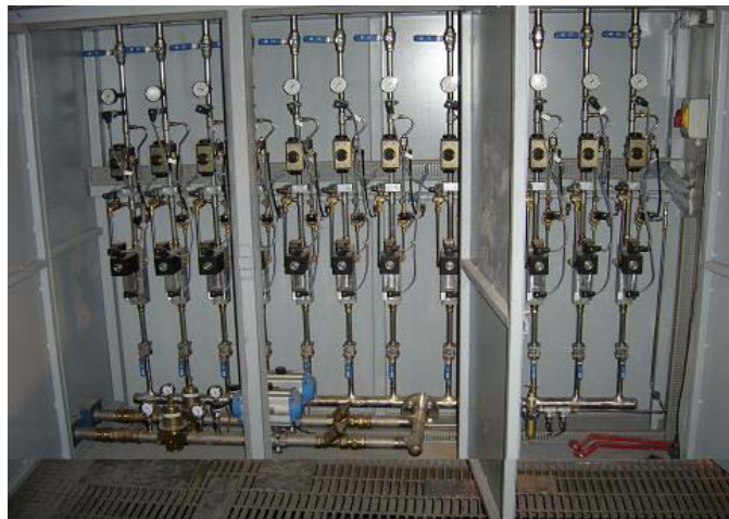
Figure 5-3: Valve/Gas station.
