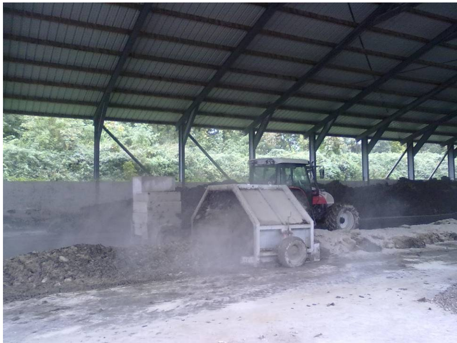
Figure 40: Stabilization Process of Drilled Material with a Turn-Over Machine 2
