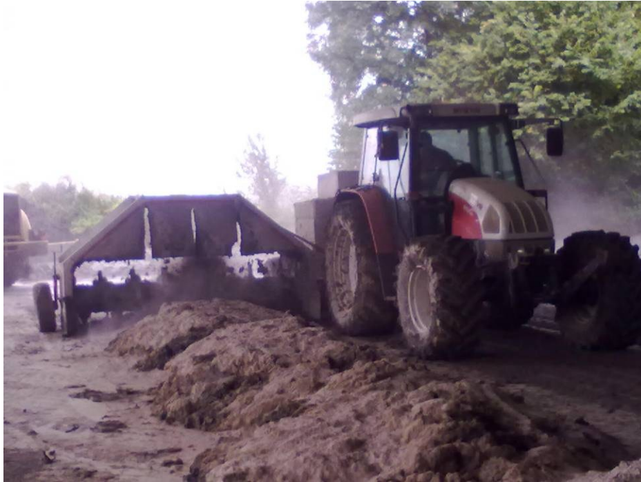
Figure 39: Stabilization Process of Drilled Material with a Turn-Over Machine 1
