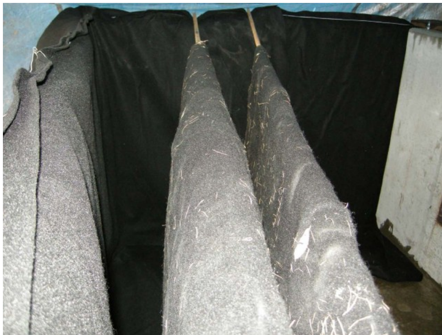
Figure 15: Multiple layers of the blasting mats
