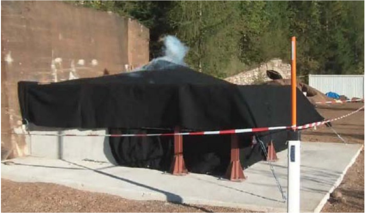
Figure 16: Blasting site during the explosion
