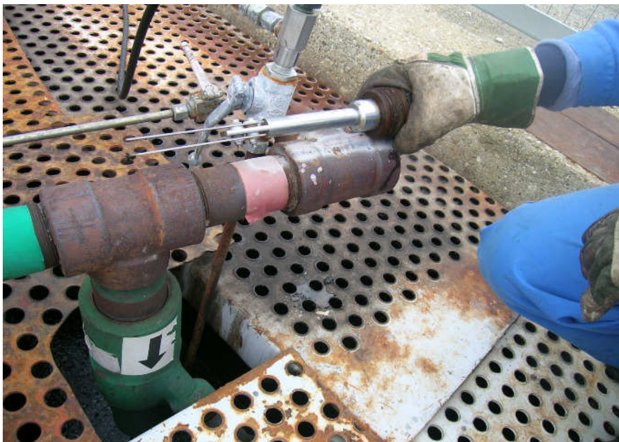
Background Data 17 – Example Picture of Surface/ Wellhead Coupons Installation of Prottes 109
