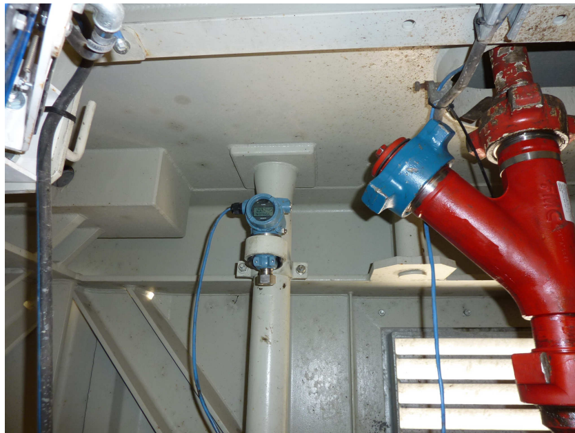
Figure 9.3 - Pressure Sensor for the cementing line - not mounted
