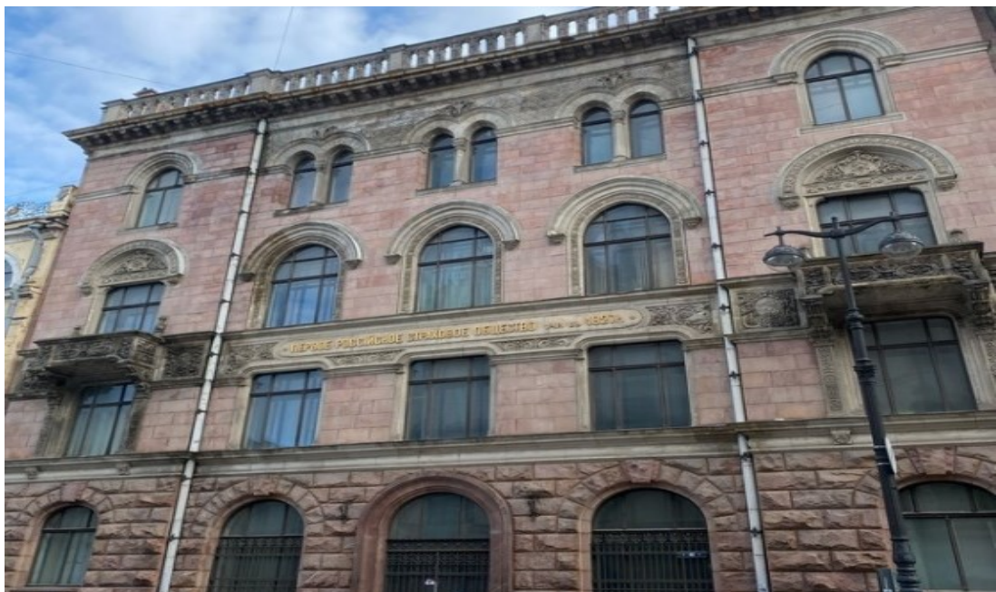
Figure 9. The house on Bolshaya Morskaya Street, 40
