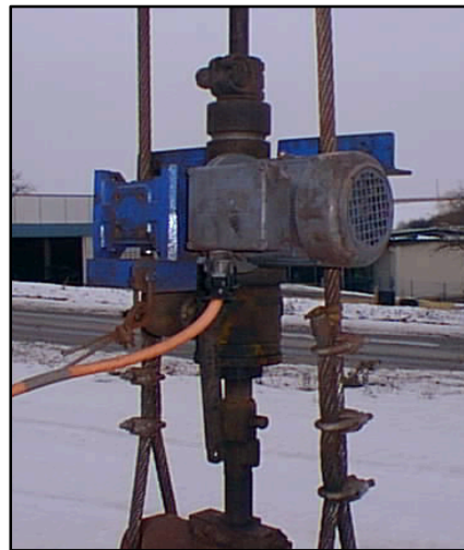
Figure 27: ECRR system installation.
