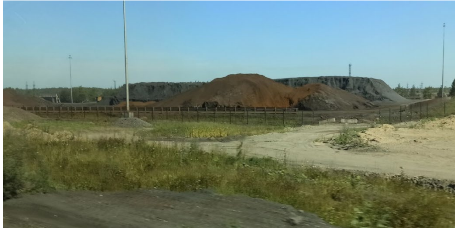
Figure 16: View of the sludge storage facility No. 2 (Yevgeny Vinogradov, 2021)
