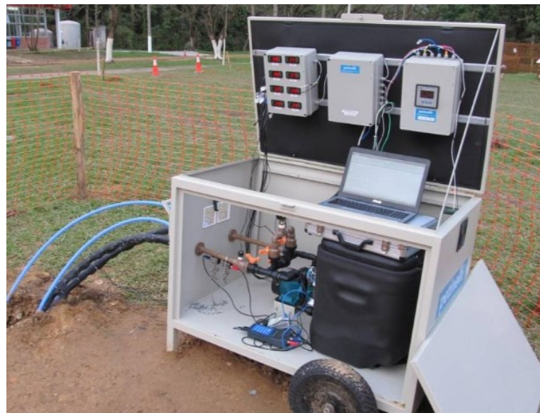
Figure 53: Geothermal response test 295
