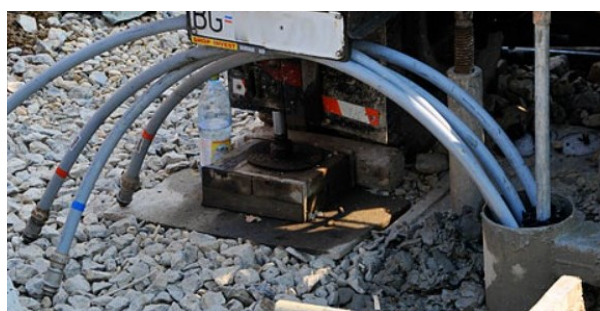
Figure 29: Installation of a geothermal probe 96
