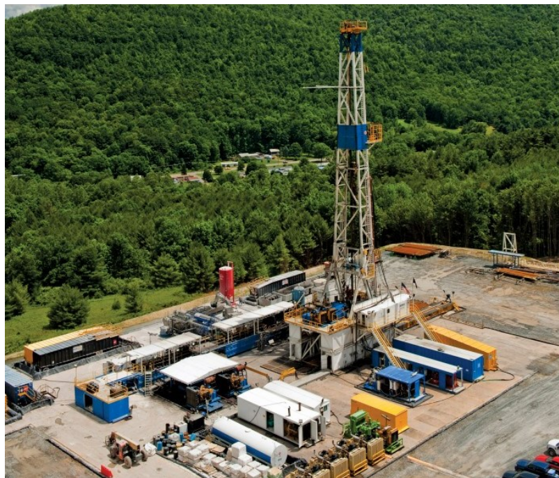
Figure 30: Rotary drilling rig 99
