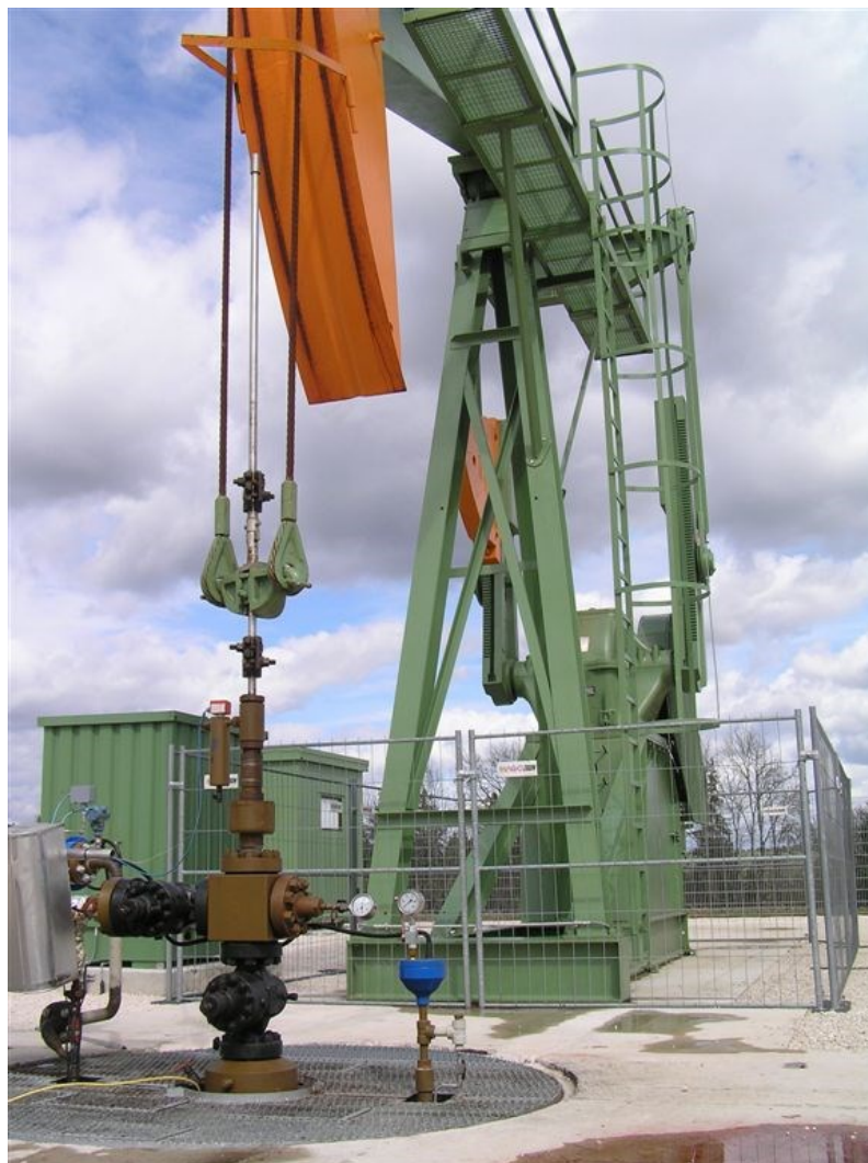
Figure 32: Murag surface installation
