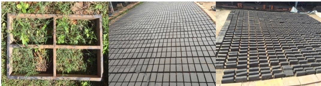
Figure 22: Molding and drying of the green artisanal solid bricks
