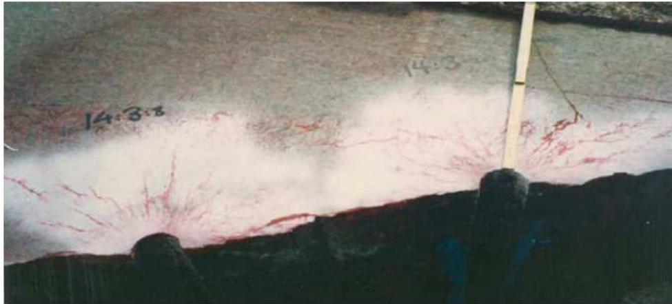
Figure I.7: Radial cracks. Saiang (2008).
