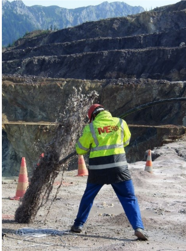
Figure 53: Draining a water filled borehole with compressed air
