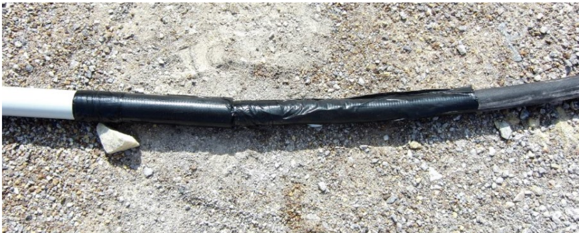
Figure 54: Connection of the charging hose with the prototype
