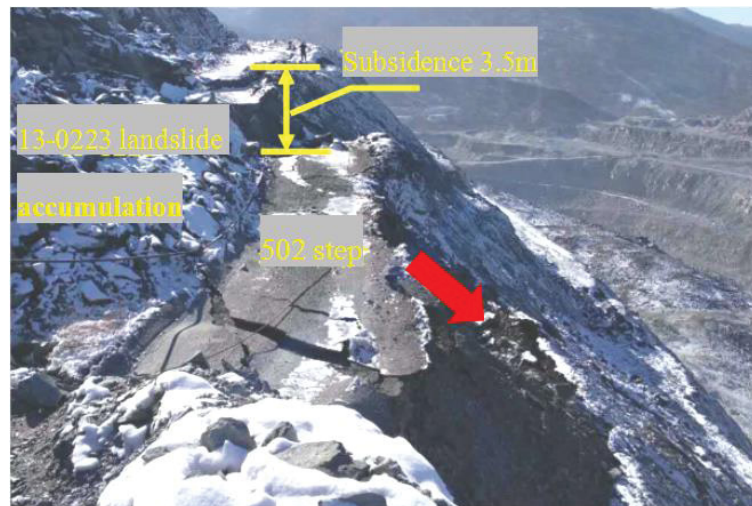
Fig.3.3 Characteristics of the top of “2016-1101” landslide
