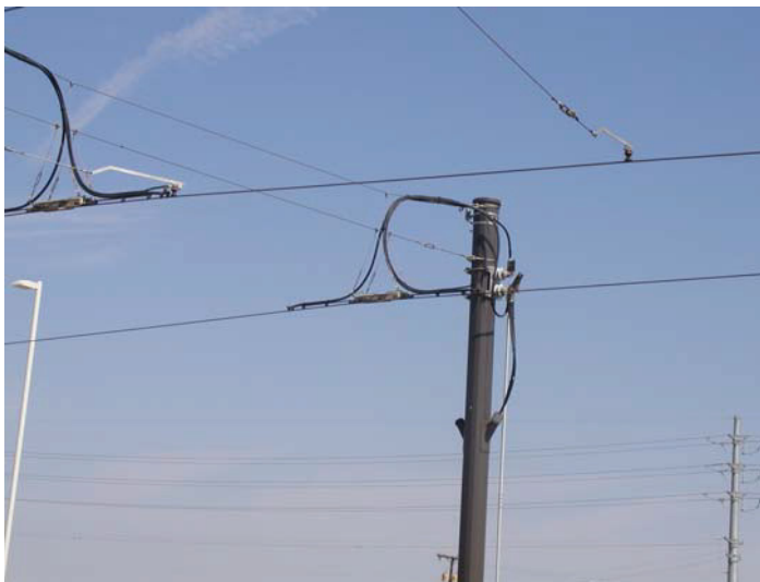
Figure 6-16 Feeder on contact line*
