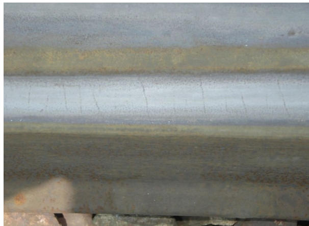
Figure 1. A crossing nose with RCF cracks. With a longitudinal slip, they are perpendicular to the running direction of the wheel.
