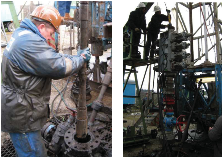
Figure 31: Left: Insertion of the deflector shoe into the tubing head; Right: Tubing head with flanges, drilling spools, gate valve and preventer.
