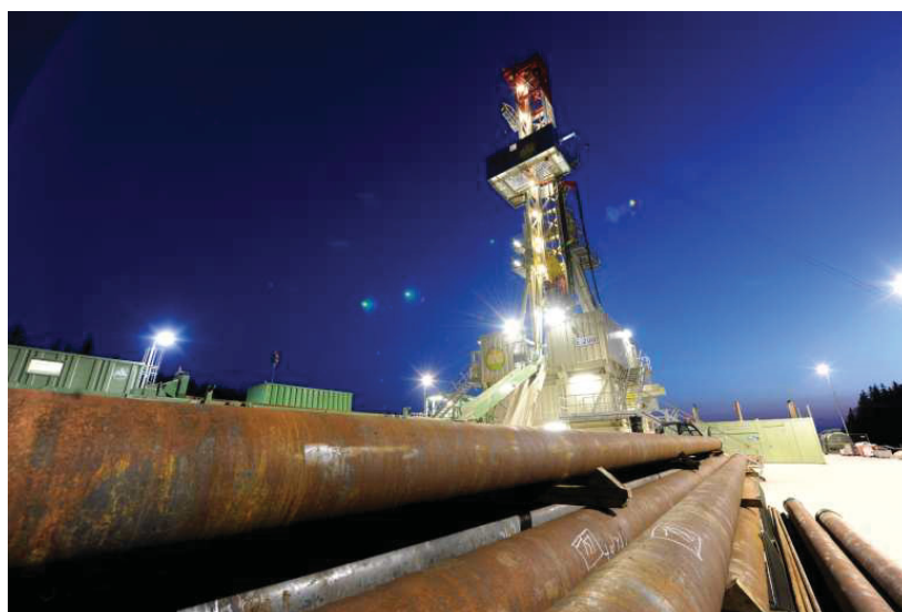
Figure 5: Drilling Rig E200 [3]
