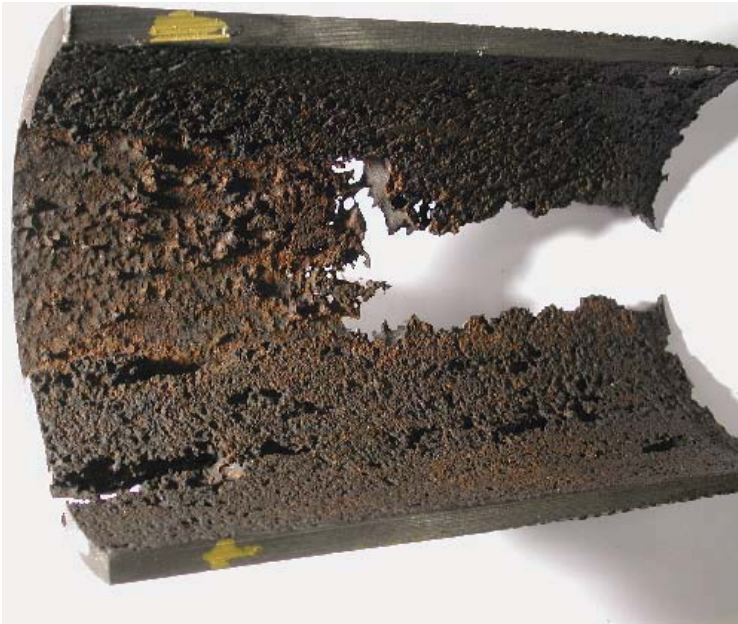
Fig. 66 PUP joint in well E-4 failed due to severe mesa corrosion
