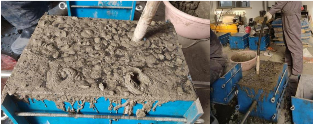
Figure 8 The process of vibrating concrete
