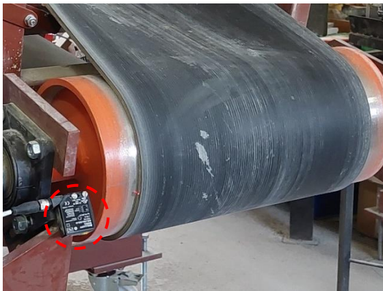
Laser sensor for measuring the belt position at the drive pulley
