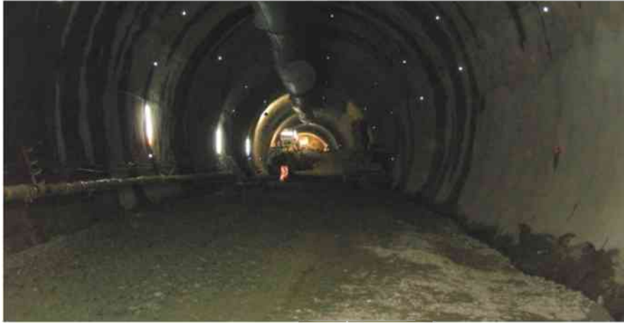
Abb. 6-100: Stein West: Fahrbahn
