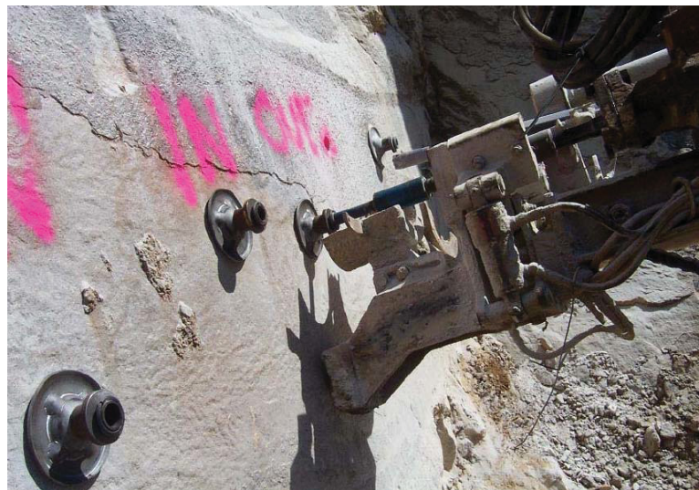
Figure 61: Installation of Ezi Bolt [49]
