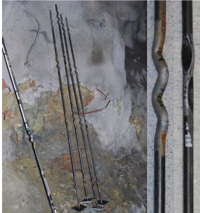
Figure 79: D-Bolt and anchor alternatives [63]
