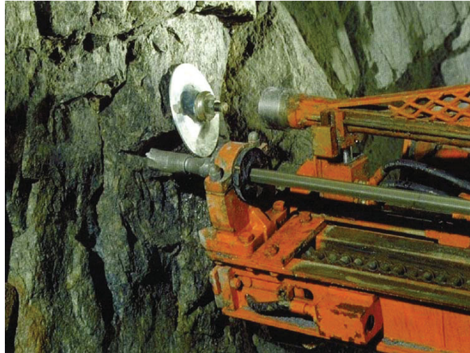
Figure 28: Mechanized rock bolter for CT-Bolt installation [33]
