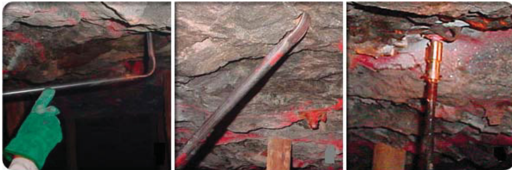
Figure 76: RS bolt during installation [61]
