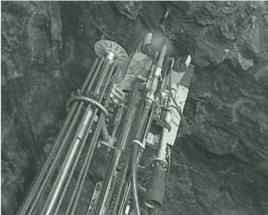
Figure 96: injection of the resin cartridge into the Borehole [73]
