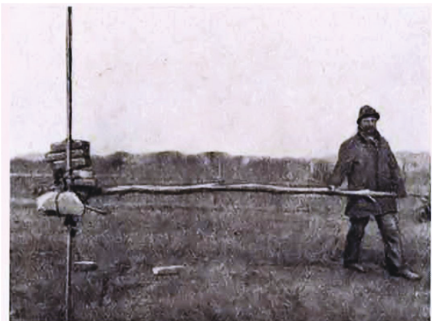
Fig. 2: Jan Medlen (1910) drills for gas. From Pois (1933).
