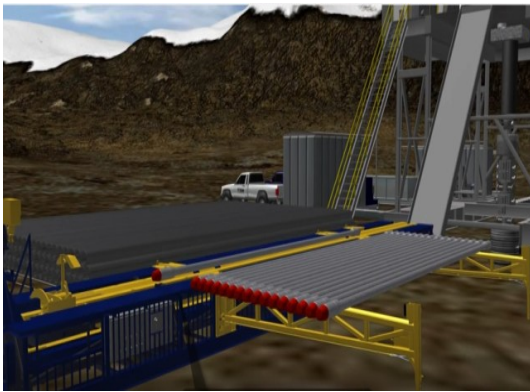
Pipe is placed on catwalk
