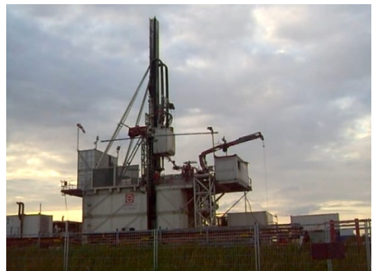
Lay down pipe
