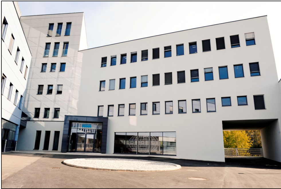
Figure 24: Office Sandvik Mining and Construction Materials Handling in Austria-Leoben 148
